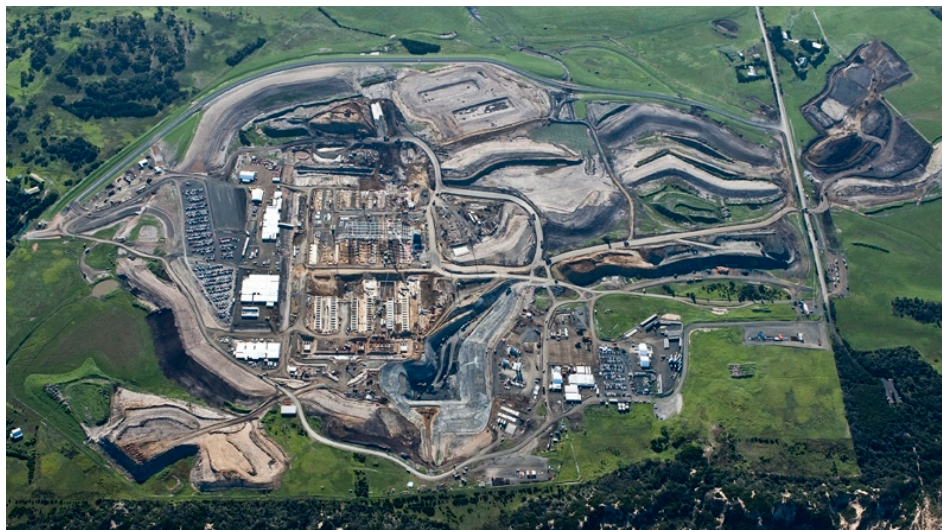
Aerial view of desalination plant
